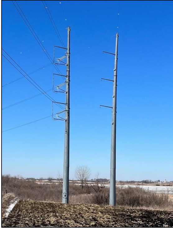
Figure 2.5-4 Typical Configuration of Two Monopole Structures Side-by-side
